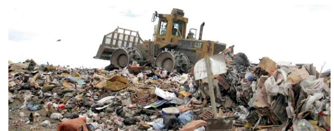
Figure 61c. Garbage is dumped in the landfill and then compacted by tractor and covered with soil. (Photos by R.Turner)
