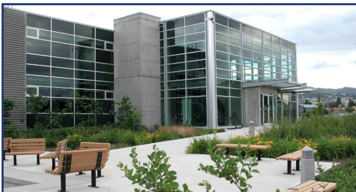
Figure 54a. City of Kamloops Centre for Water Quality, water treatment plant.
