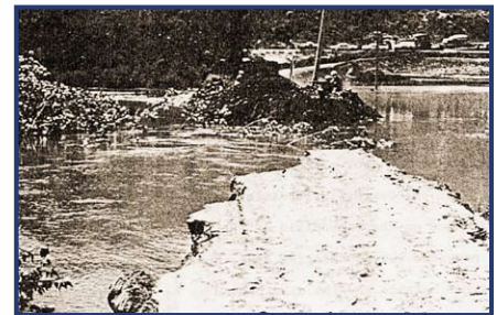
Figure 24b. Breached dyke at the Oak Hills subdivision during the flood of 1972. Photos courtesy of R. Buchanan and B. Gerath.
