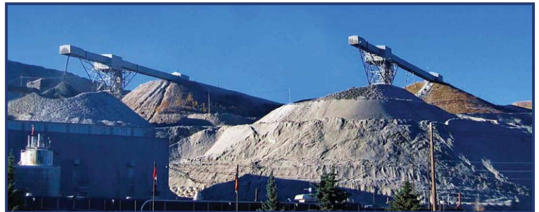
Figure 40. Conveyor belts carry football size blocks of ore from the pit to stockpiles (centre) at the mill (lower left), ready for processing. (Photo by R. Anderson)
