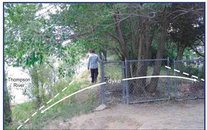
Figure 27. The integrity of this dyke on the North Shore along the Thompson River may be compromised by the trees that grow on it. Trees can weaken a dyke; when tree roots die, they leave behind small tunnels that can allow water to flow through the dyke during a flood. Such small water flows can lead to larger failure of the dyke. (Photo by R.Turner)
