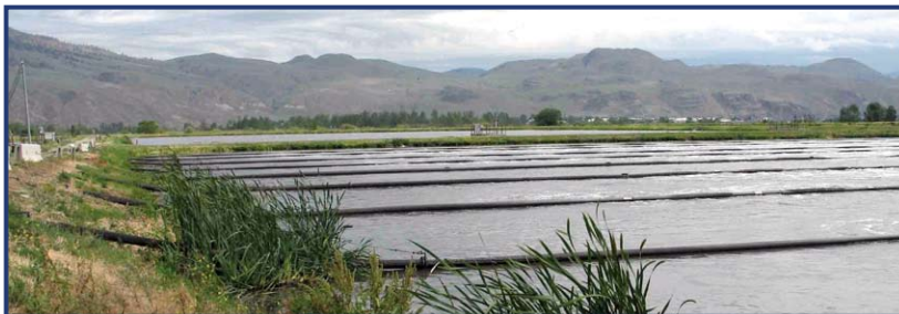
Figure 56. Bubblers within the secondary treatment lagoon mix oxygen into the wastewater. This oxygen is essential to sustain bacteria that feed on and digest the organic matter, converting organic compounds to non-harmful products. Abundant green algae on the surface and shoreline plants reflect the nutrient-rich nature of the waste water. (Photo by R..Turner)
