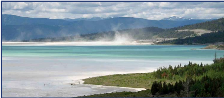
Figure 43. The tailings pond for the Highland Valley mine contains white rock mud, the waste product of the milling process. The water in the pond has an aqua blue colour due to reflection of sunlight from the white lake floor (swimming pools are painted white to create this same beautiful blue colour). When mining has ended, the tailings pond will be drained of water, and its surface covered with soil and planted with grasses to transform it into pasture or meadows for cattle or deer. (Photo by R.Turner)
