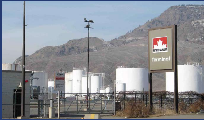
Figure 49. Bulk petroleum storage depot on Tranquille Road near the airport. Tanker trucks transport gasoline from the depot to gas stations from Merritt to Williams Lake in the BC Interior. The depot is adjacent to the Trans Mountain Pipeline. (Photo by R.Turner)
